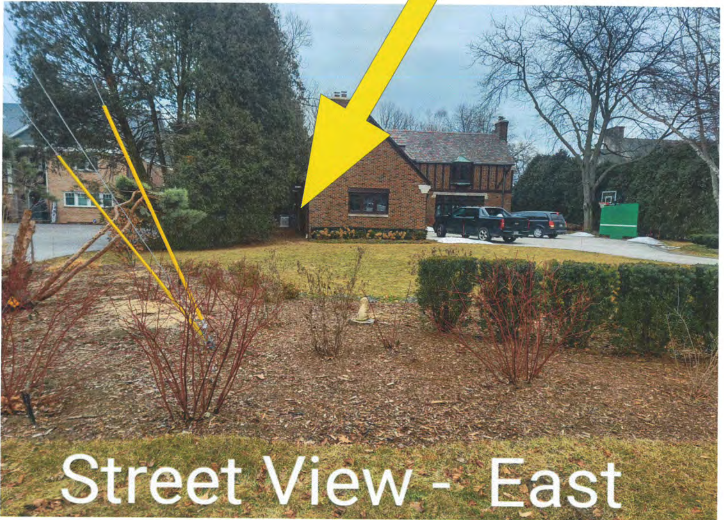
NW side- East view
