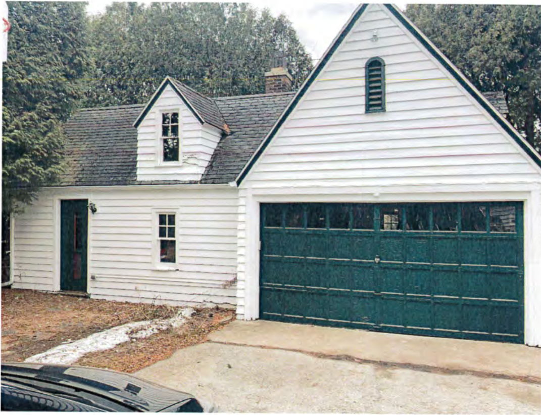
Existing Garage - East Elevation
