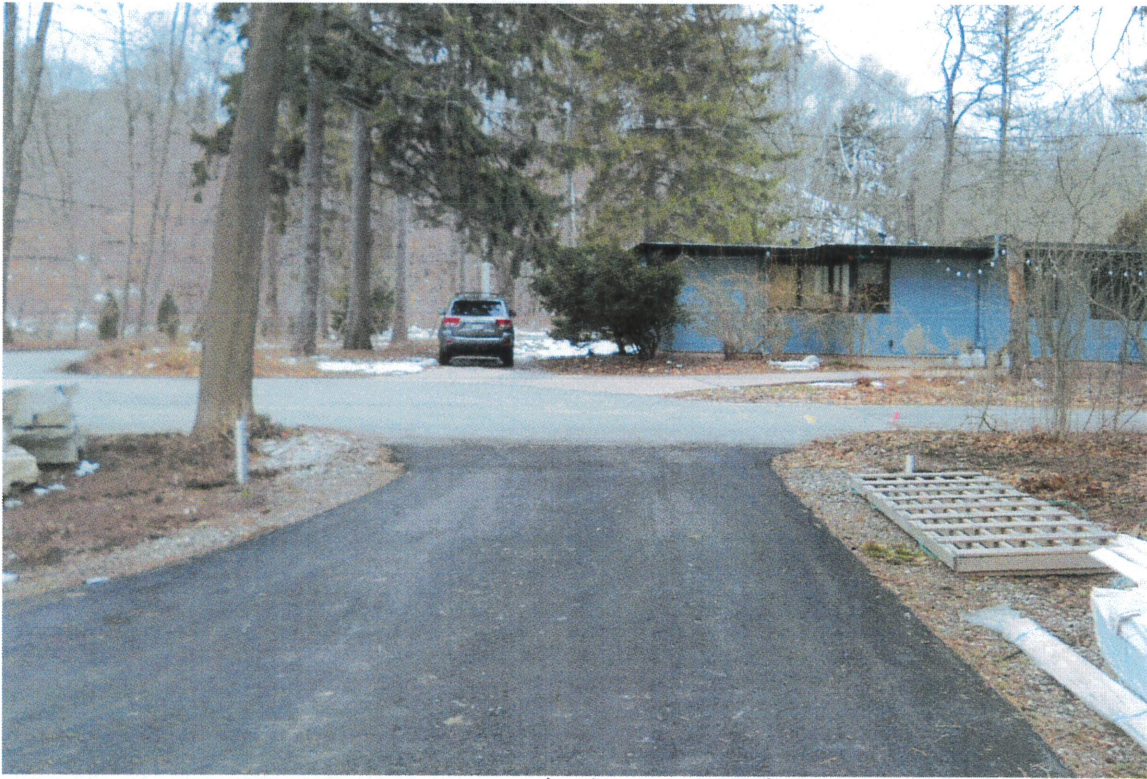
Entry area looking west
