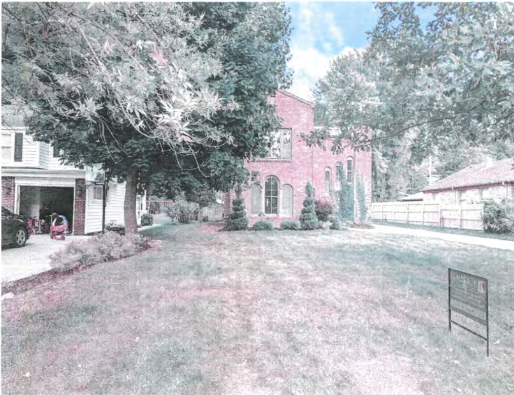
View from the front of the house, looking towards the side with the air conditioner. It is mostly hidden behind the chimney
