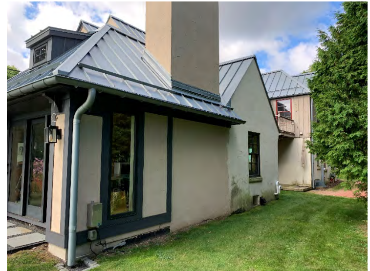
VIEW FROM THE NORTHEAST
