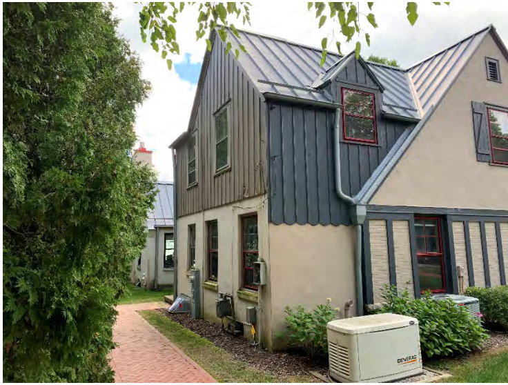
VIEW FROM THE NORTHWEST
