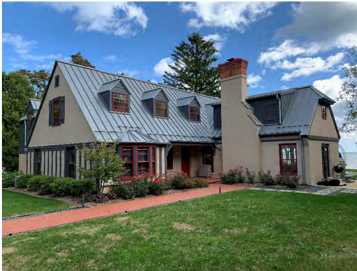
VIEW FROM THE SOUTHWEST
