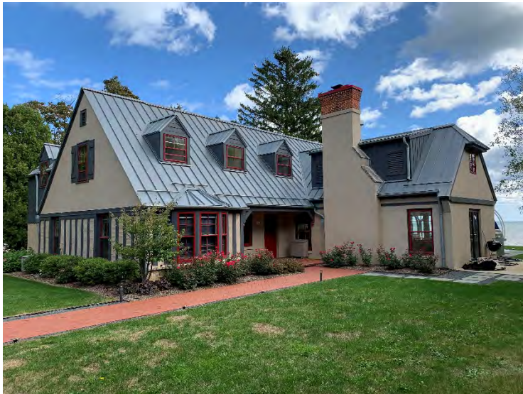
VIEW FROM THE SOUTHWEST
