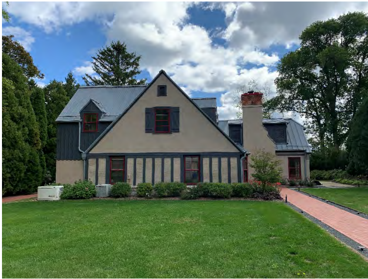
VIEW FROM THE WEST
