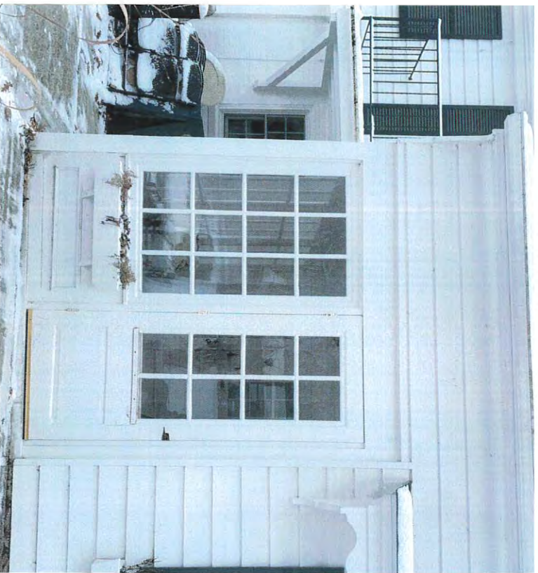
Mudroom: North facing wall; CURRENT
