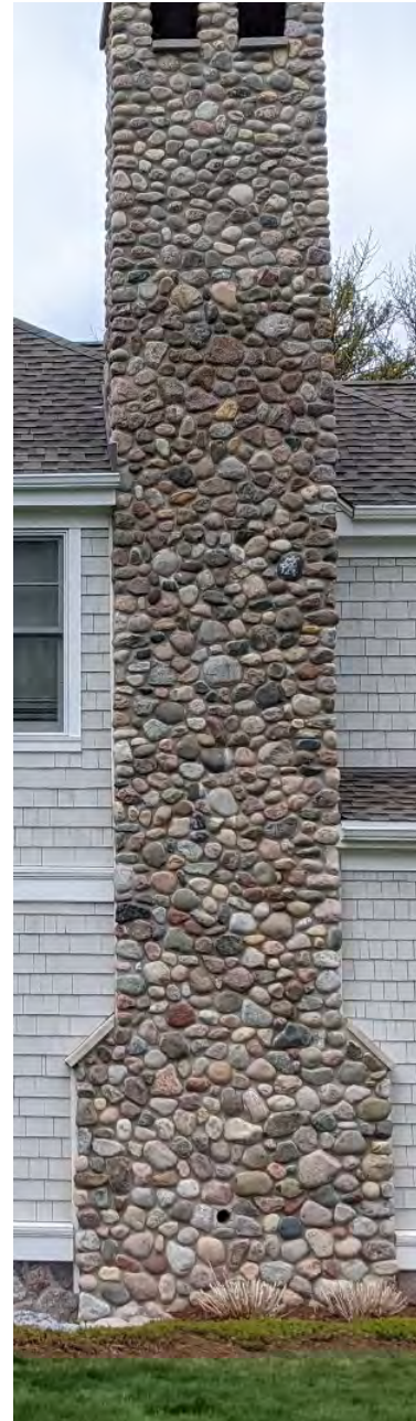
Stone Veneer - Chimney Fieldstone similar to Residence
