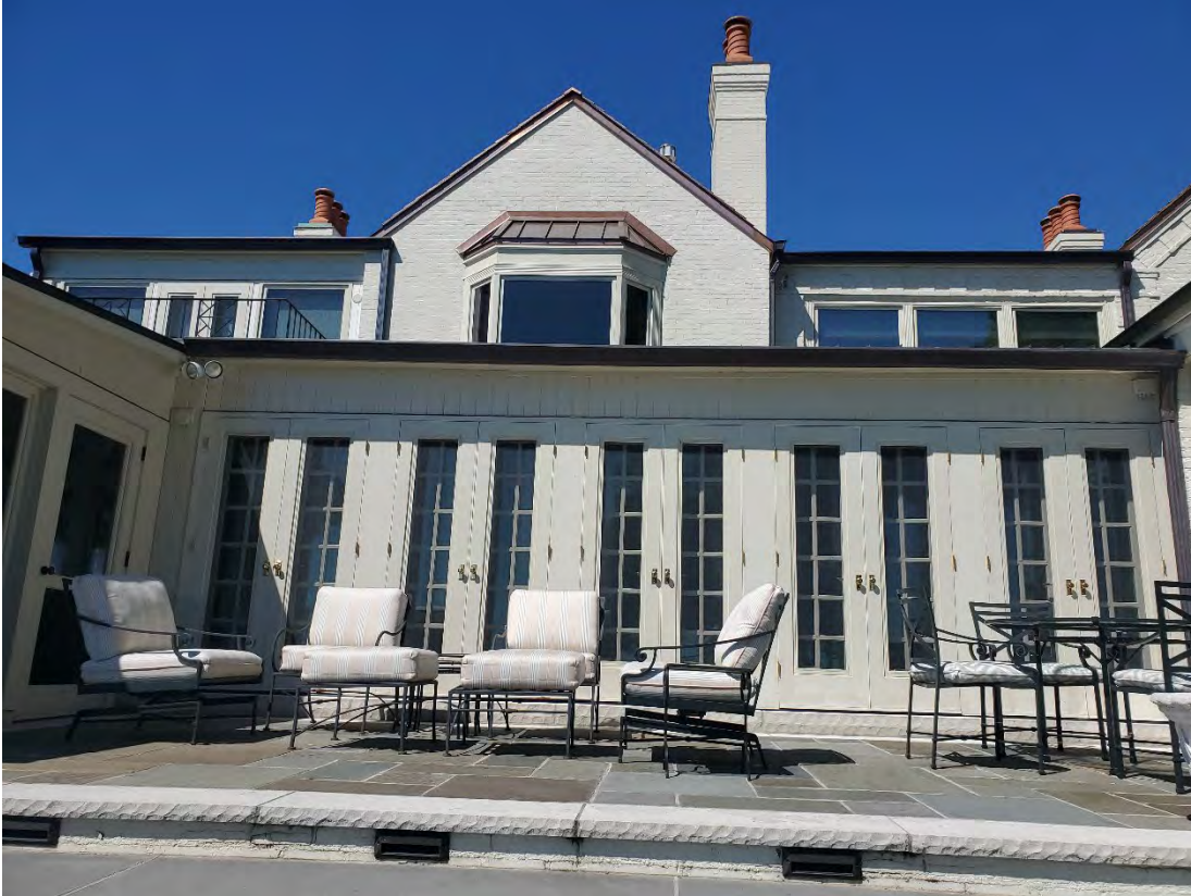
Existing Uncovered Rear Porch (Proposed location of new roof) – View Looking West
