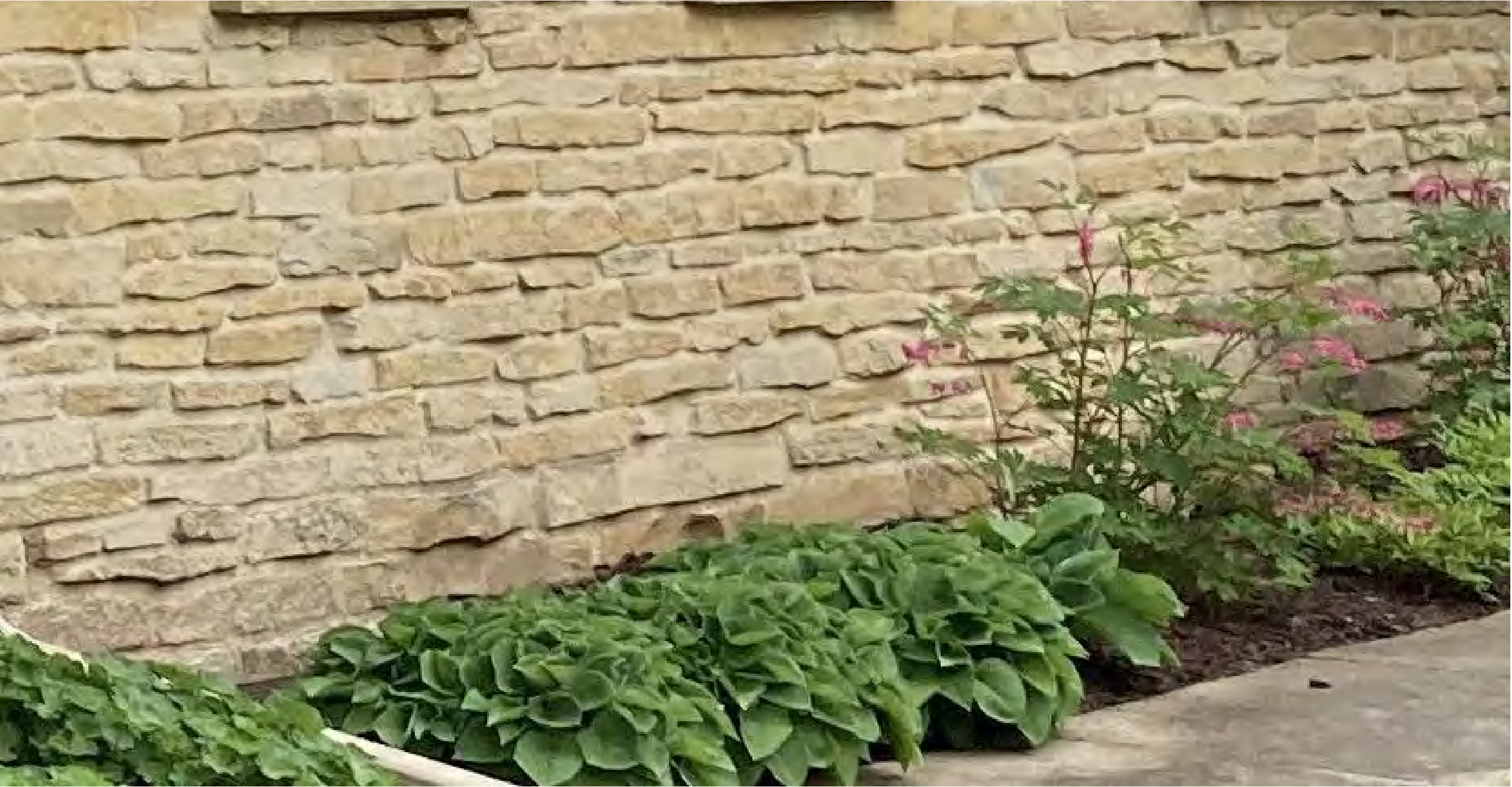
MASONRY: Reuse salvage Limestone from demo to patch as needed (Same as Existing)
