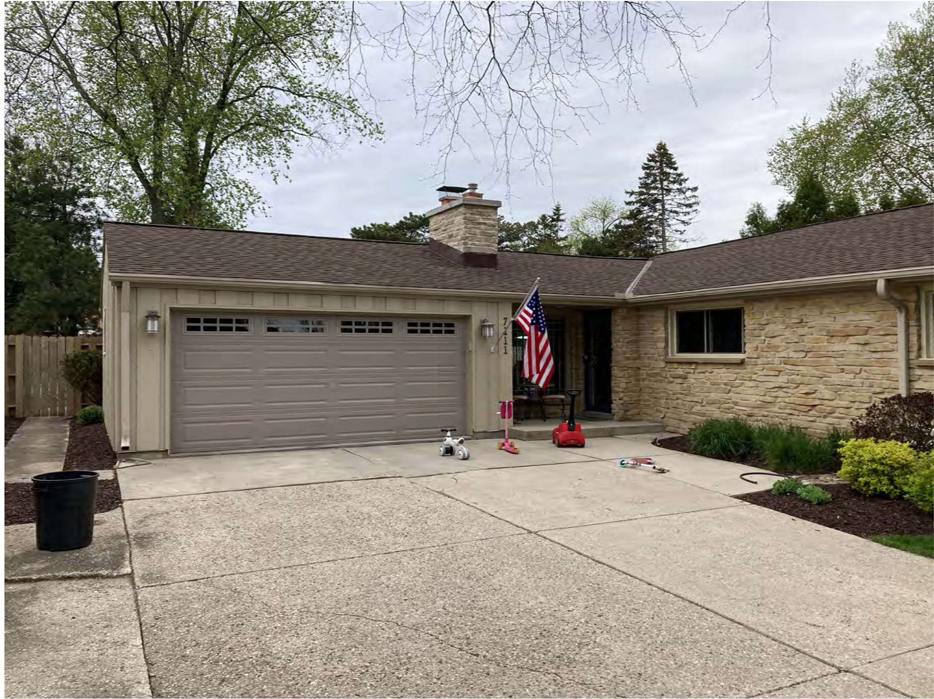
2 | EXISTING EXTERIOR - SOUTHEAST ELEVATION
