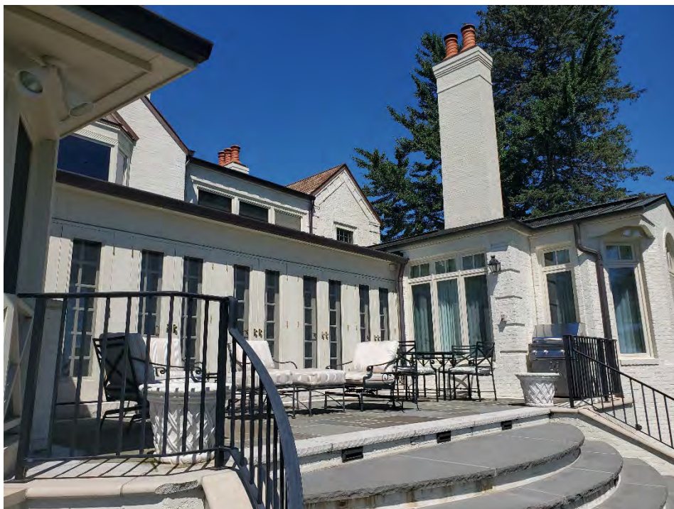
Rear Elevation – Looking Northeast
