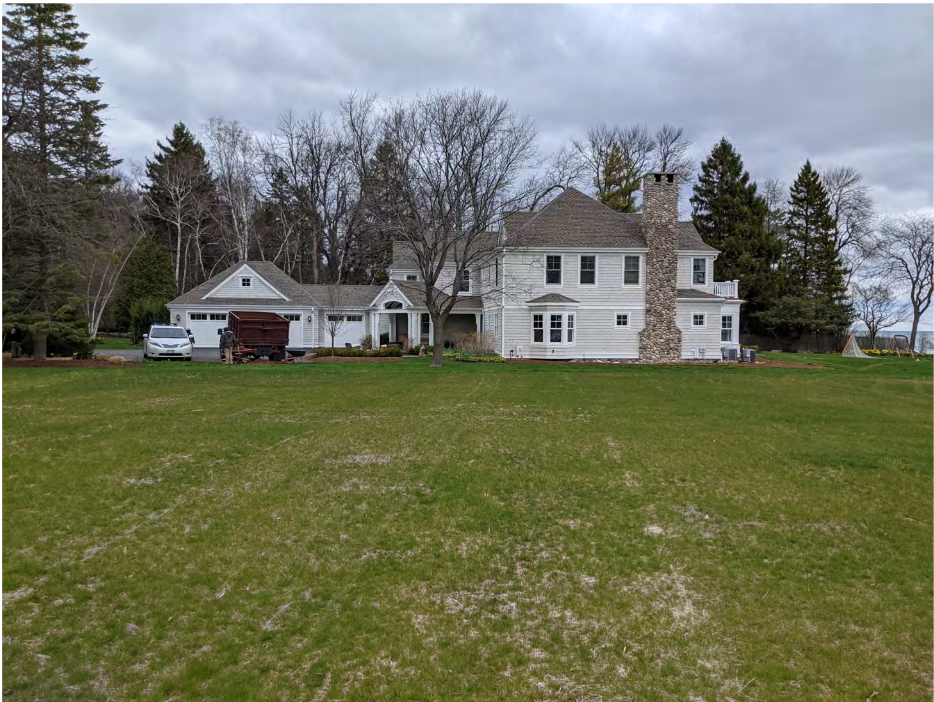
2 NORTH FACING EXISTING PROPERTY
