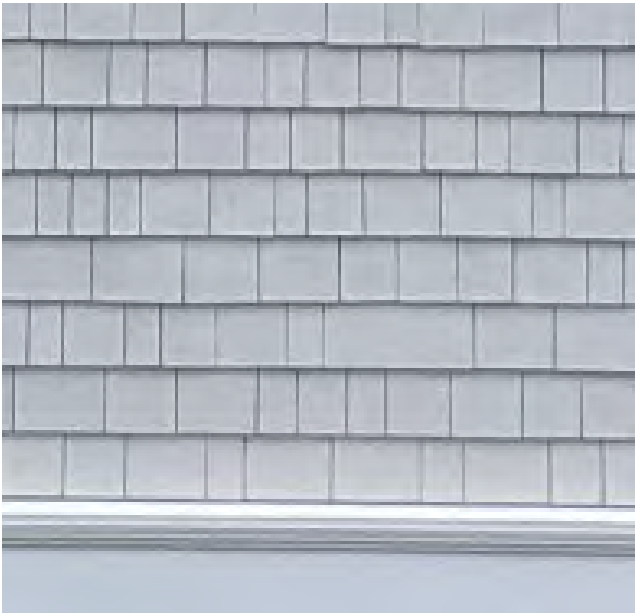
Cedar Wall Shingle – 6” Exposure / Random width / alternated laced outside corners Benjamin Moore – Ice Formations
