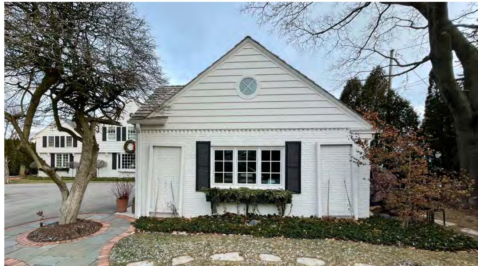
9 Front Yard, Garage Elevation
