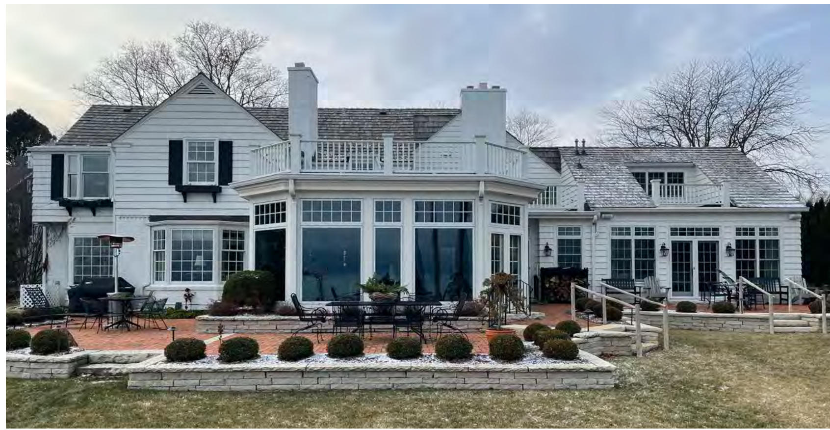
4 Backyard Looking West
