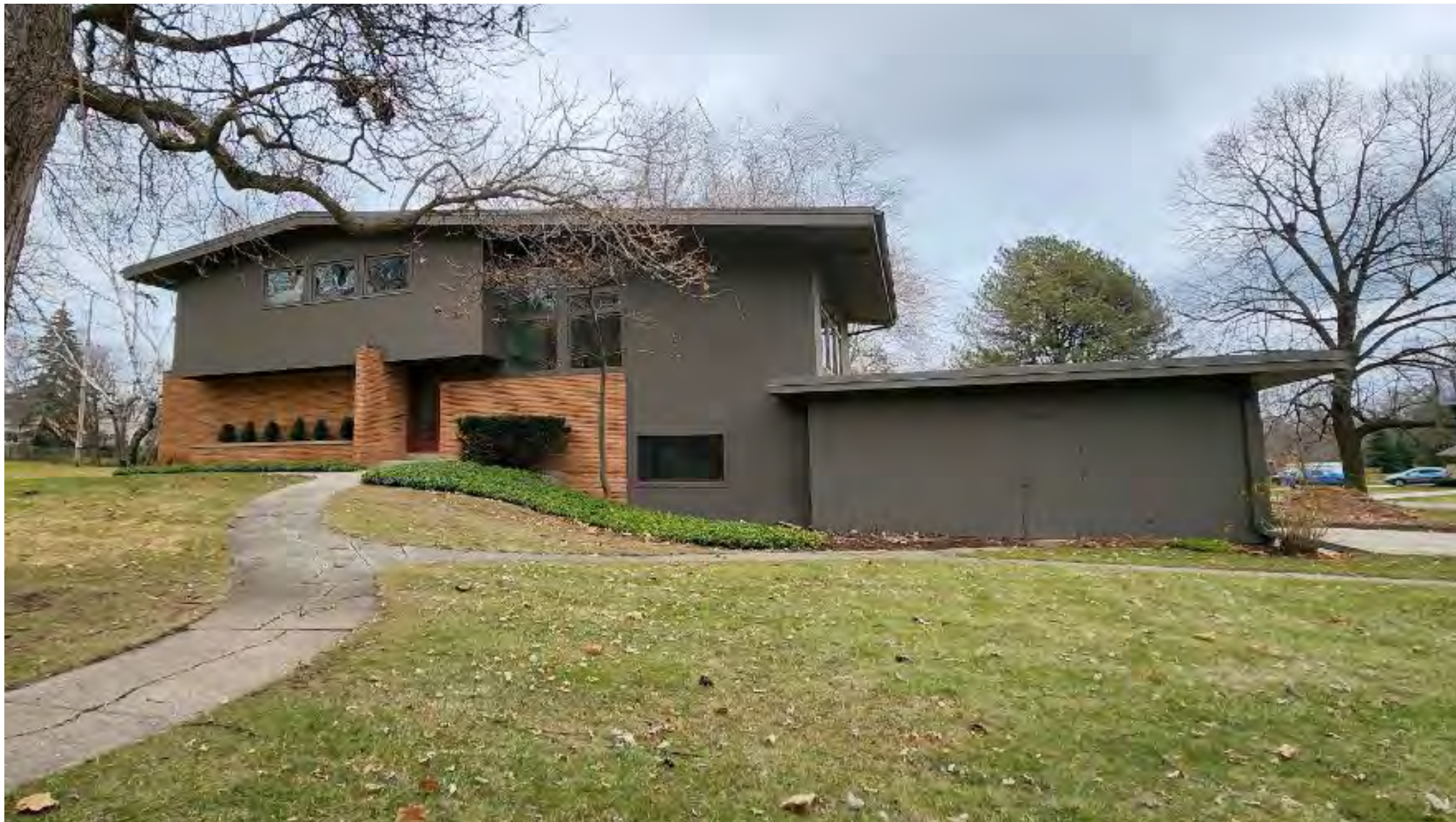
EXISTING FRONT - WEST facing Regent
