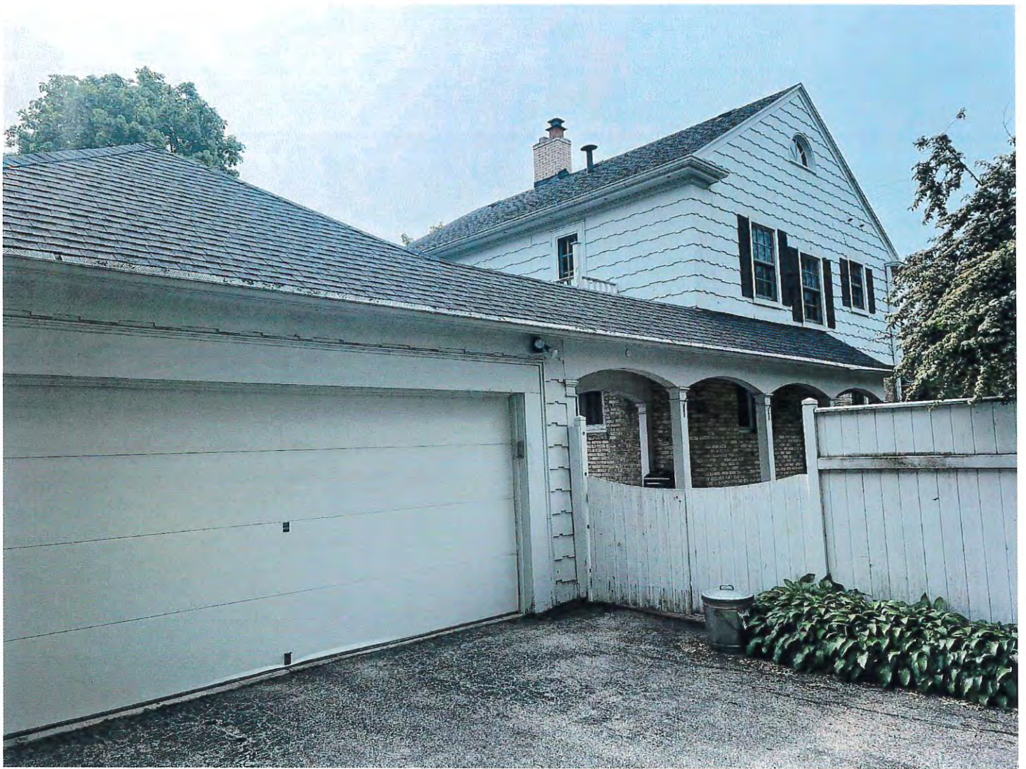
Face of garage on west side of house
