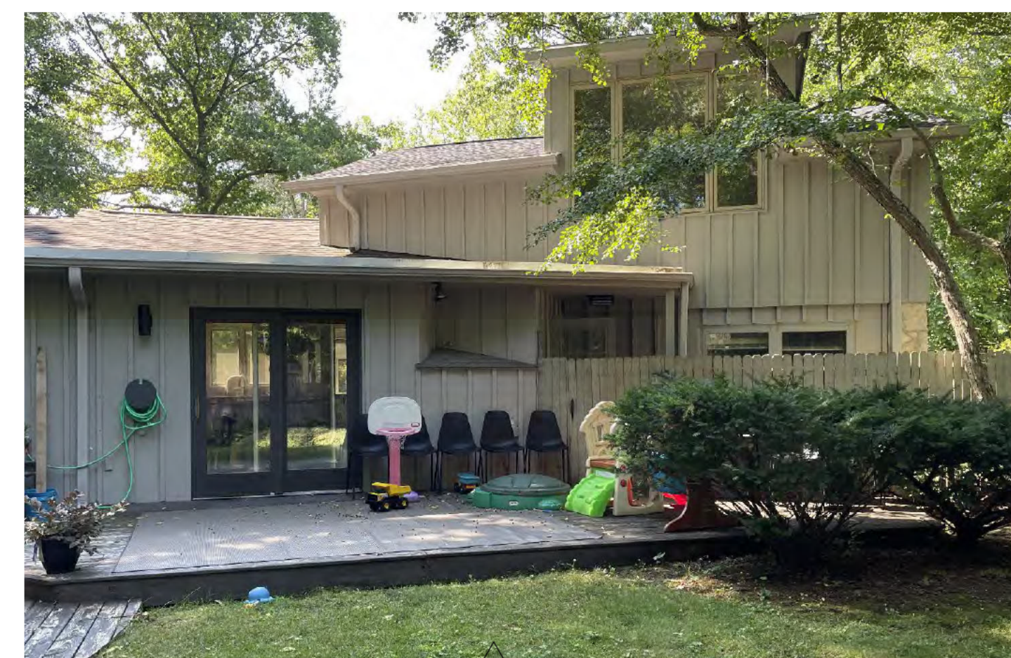
EXISTING REAR NORTH FACE @ KITCHEN DOOR PHOTO
