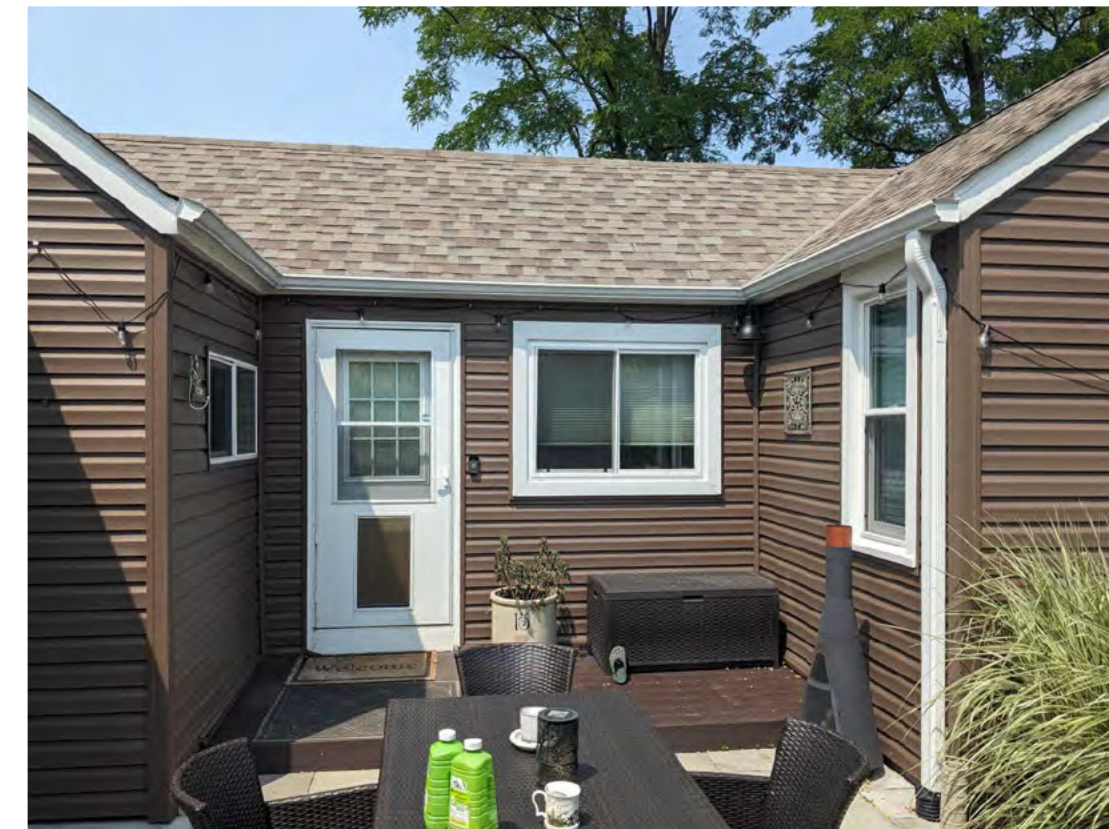
8 - S SOUTH ELEVATION, CENTER OF HOUSE
