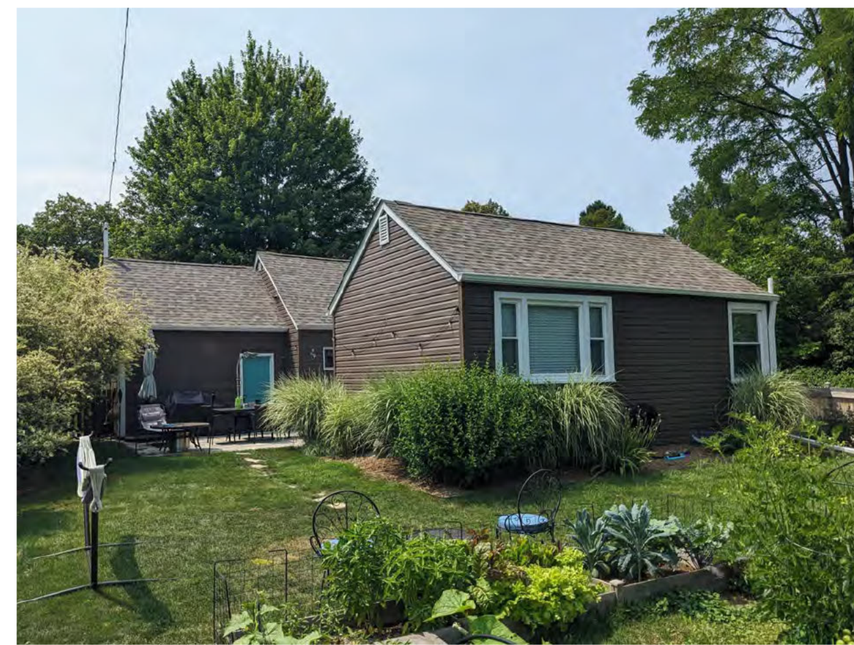
9 - SE REAR SOUTHEAST CORNER
