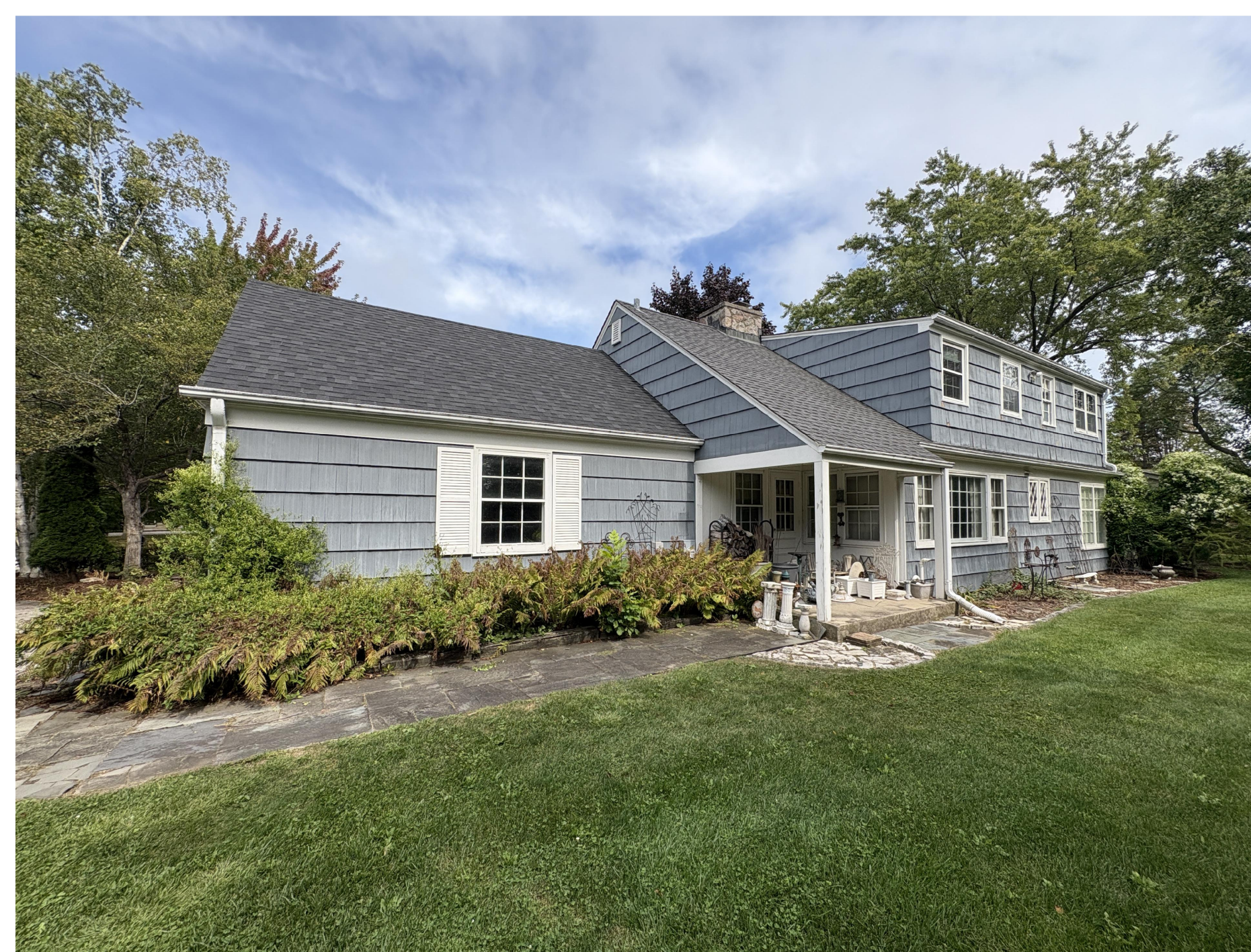
5 | EXISTING EXTERIOR - WEST
