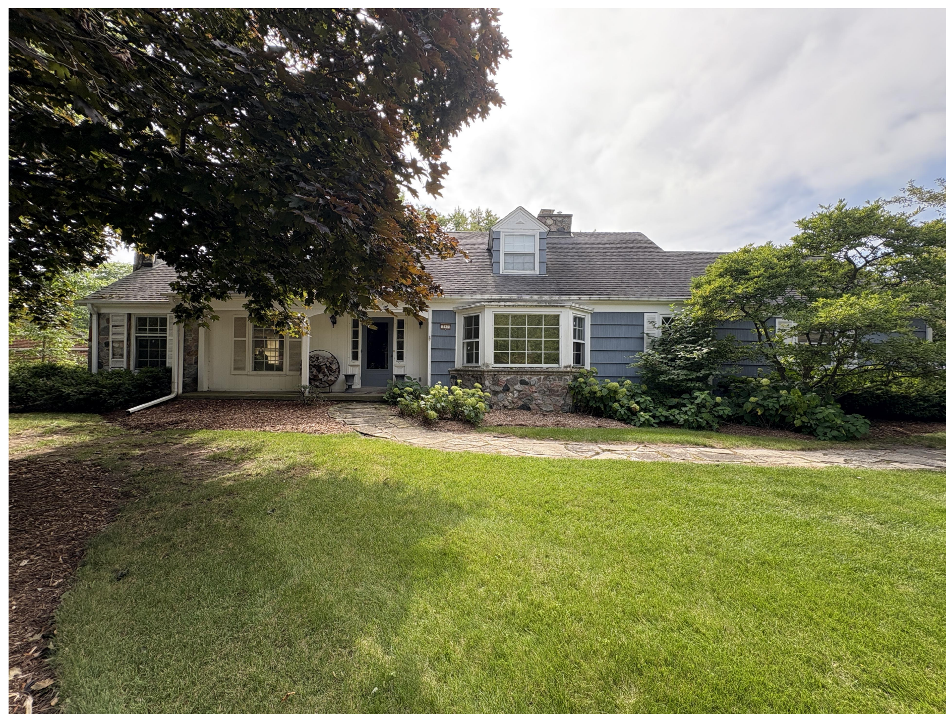
1 | EXISTING EXTERIOR - EAST
