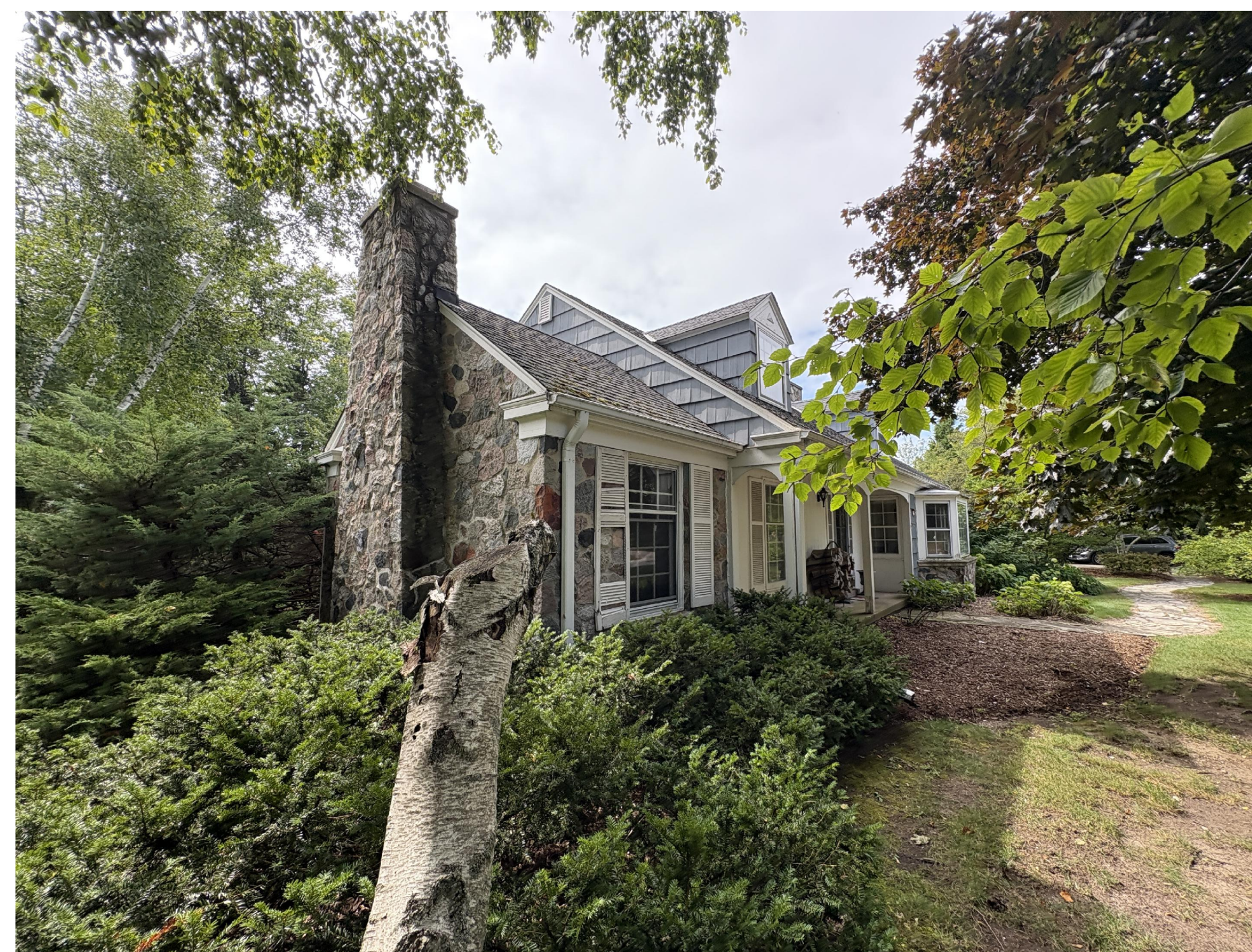
2 | EXISTING EXTERIOR - SOUTH
