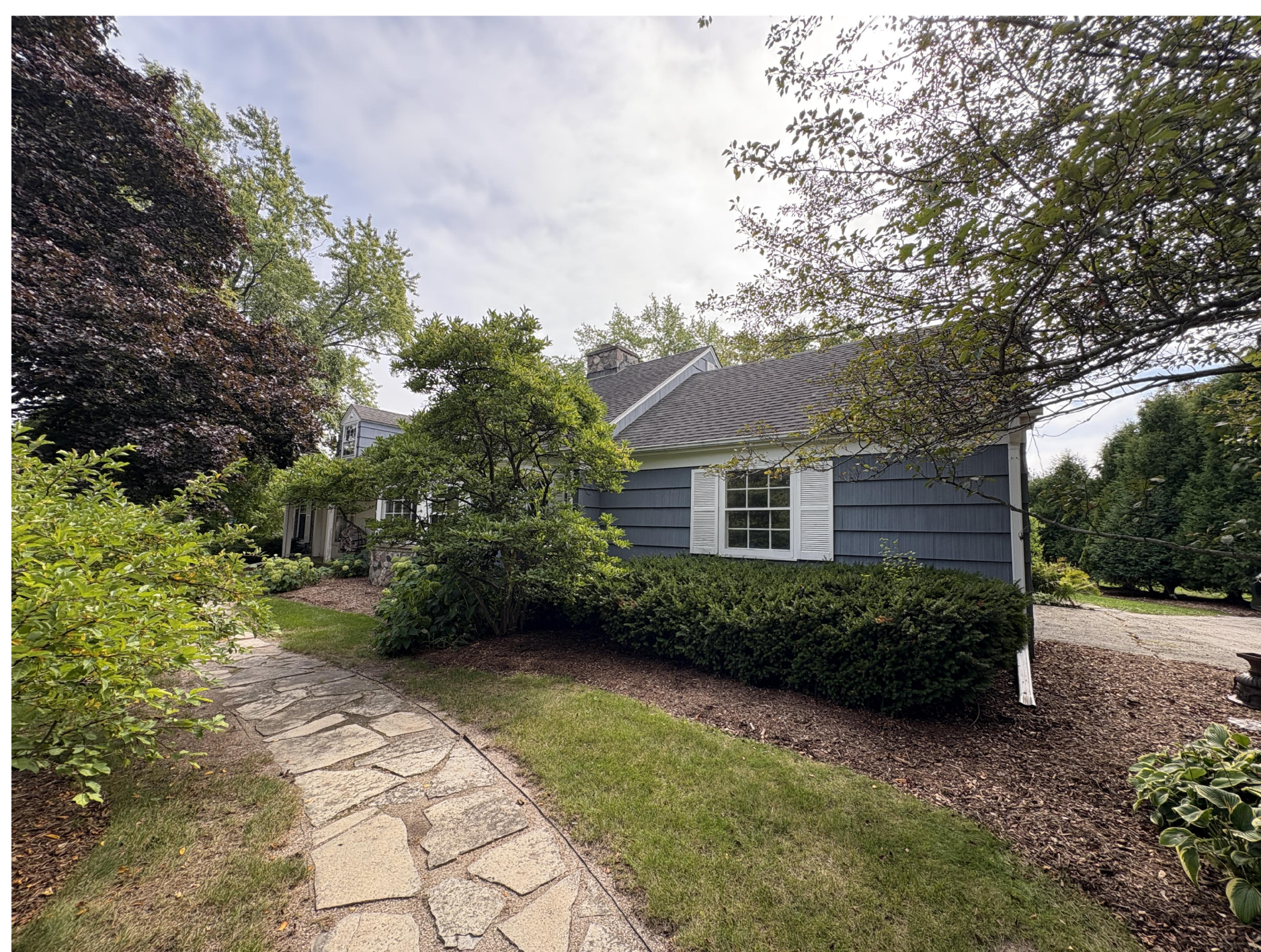
4 | EXISTING EXTERIOR - EAST
