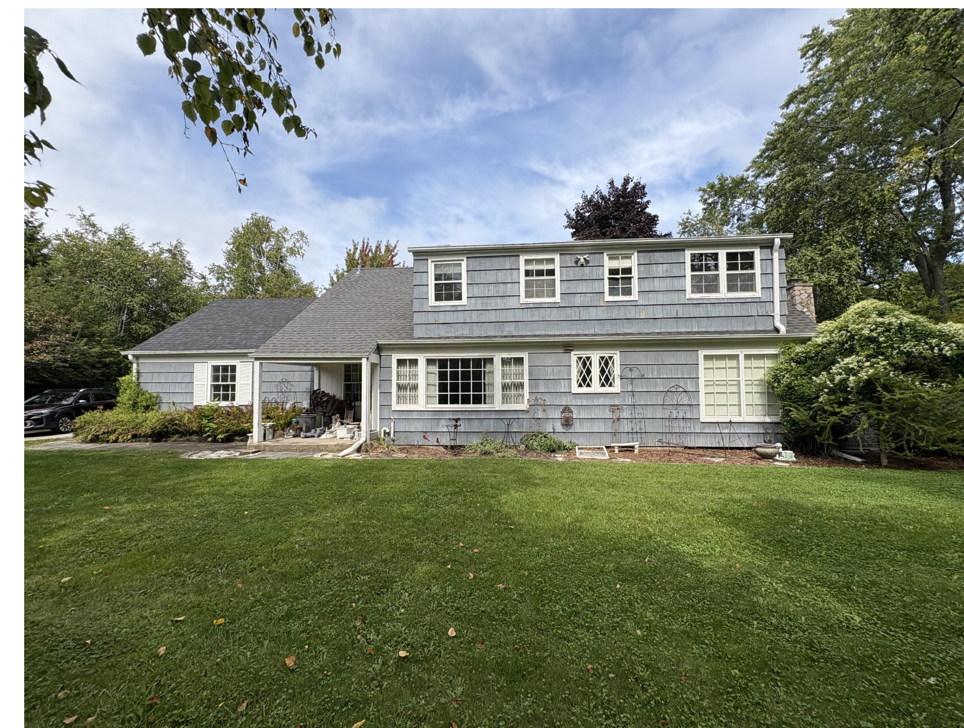
3 | EXISTING EXTERIOR - WEST
