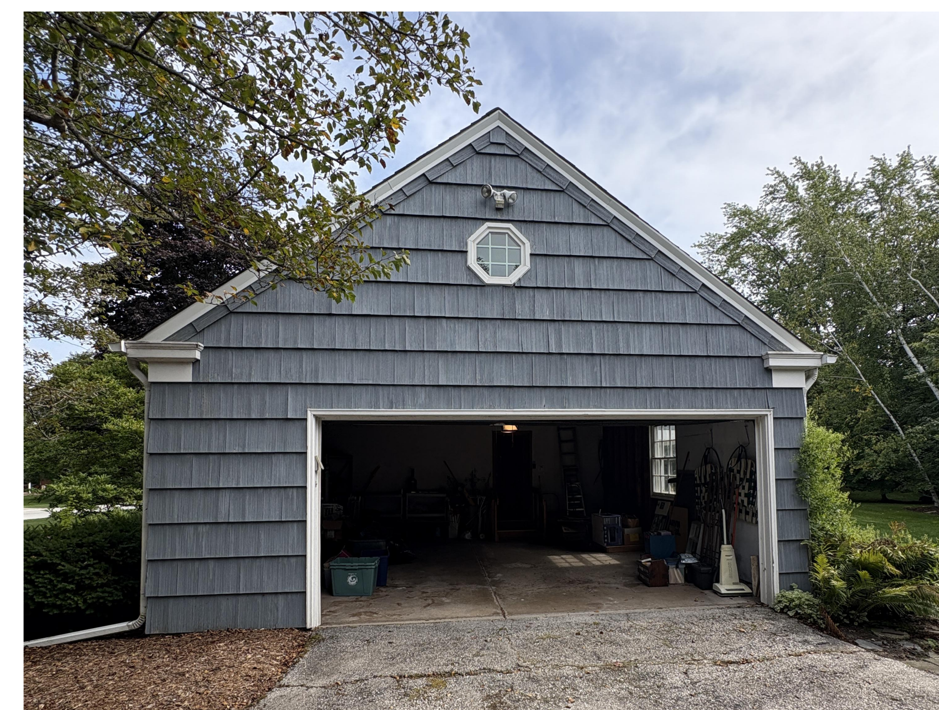
6 | EXISTING EXTERIOR - NORTH
