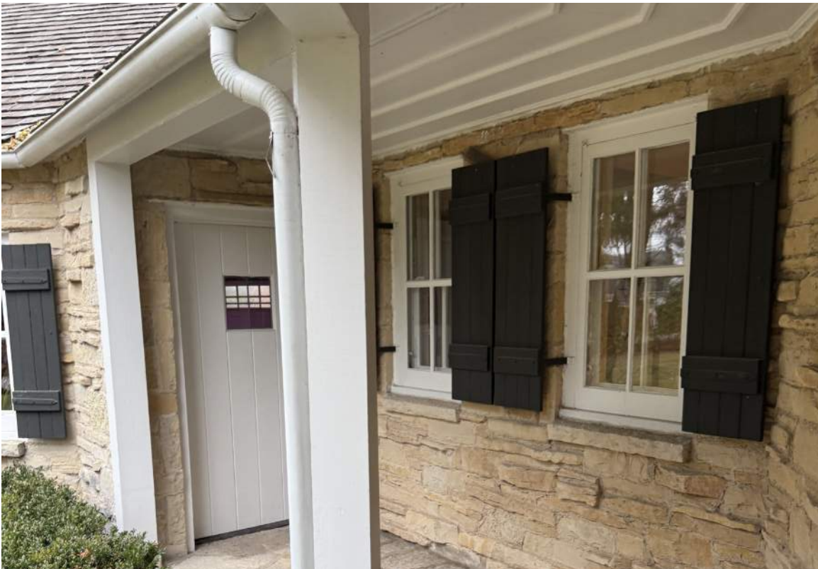
SOUTHWEST ELEVATION - PORCH AND GARAGE ENTRY
