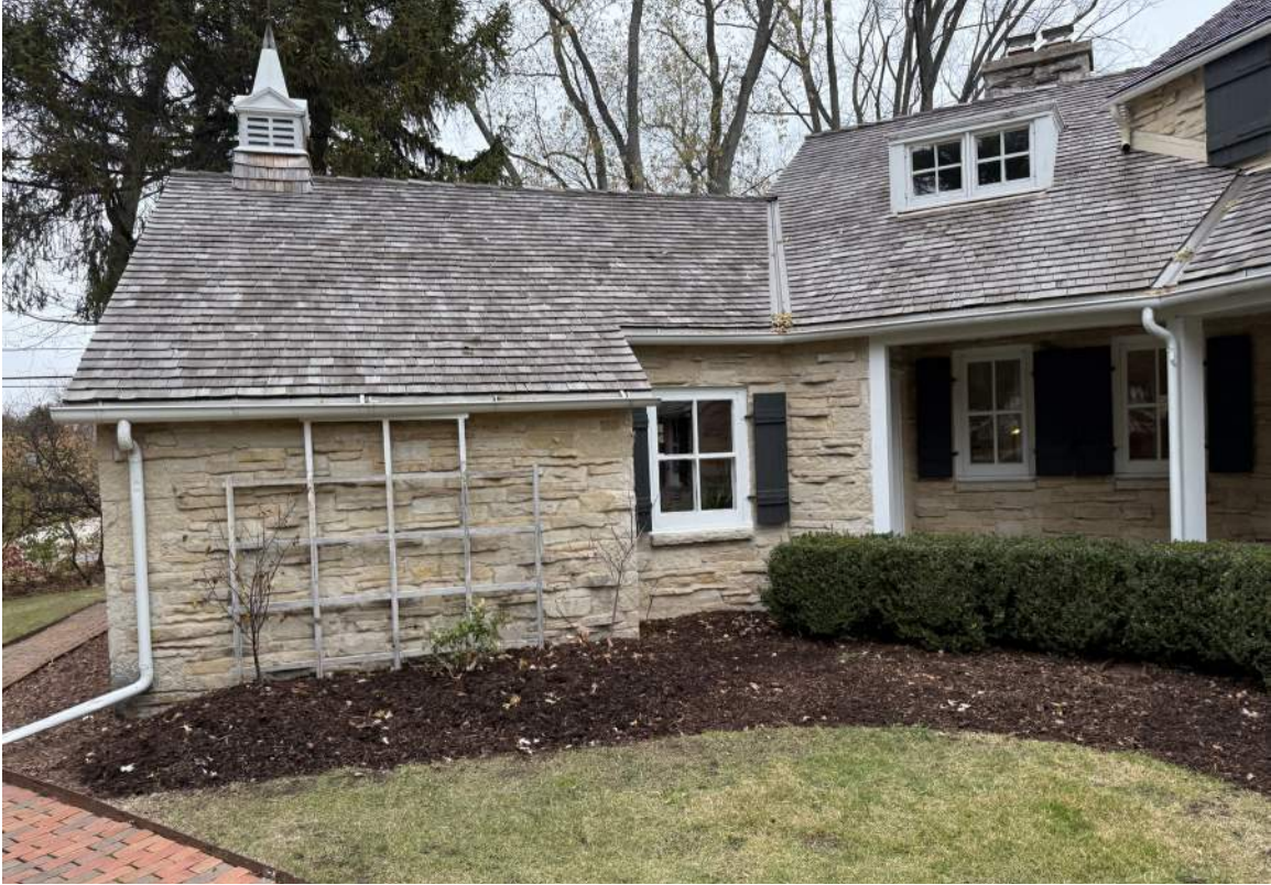
SOUTHWEST ELEVATION - GARAGE AND PORCH
