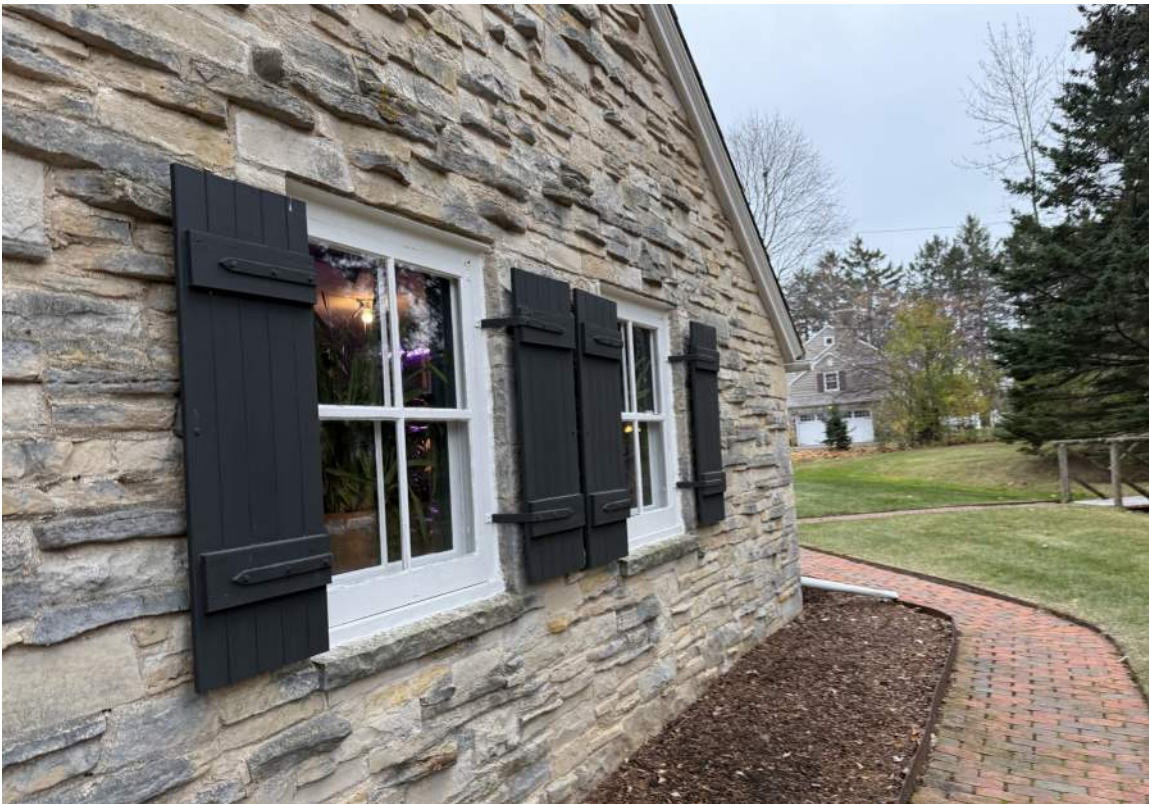
WEST ELEVATION - SIDE OF GARAGE
