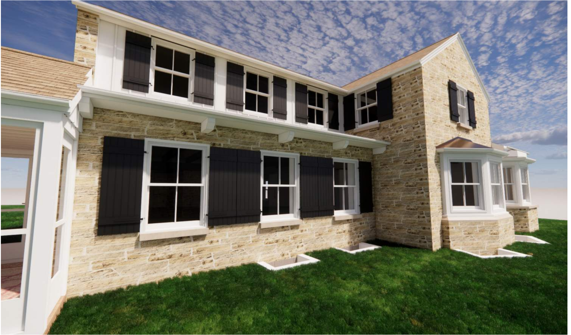
VIEW OF WEST FACADE AND BALCONY
