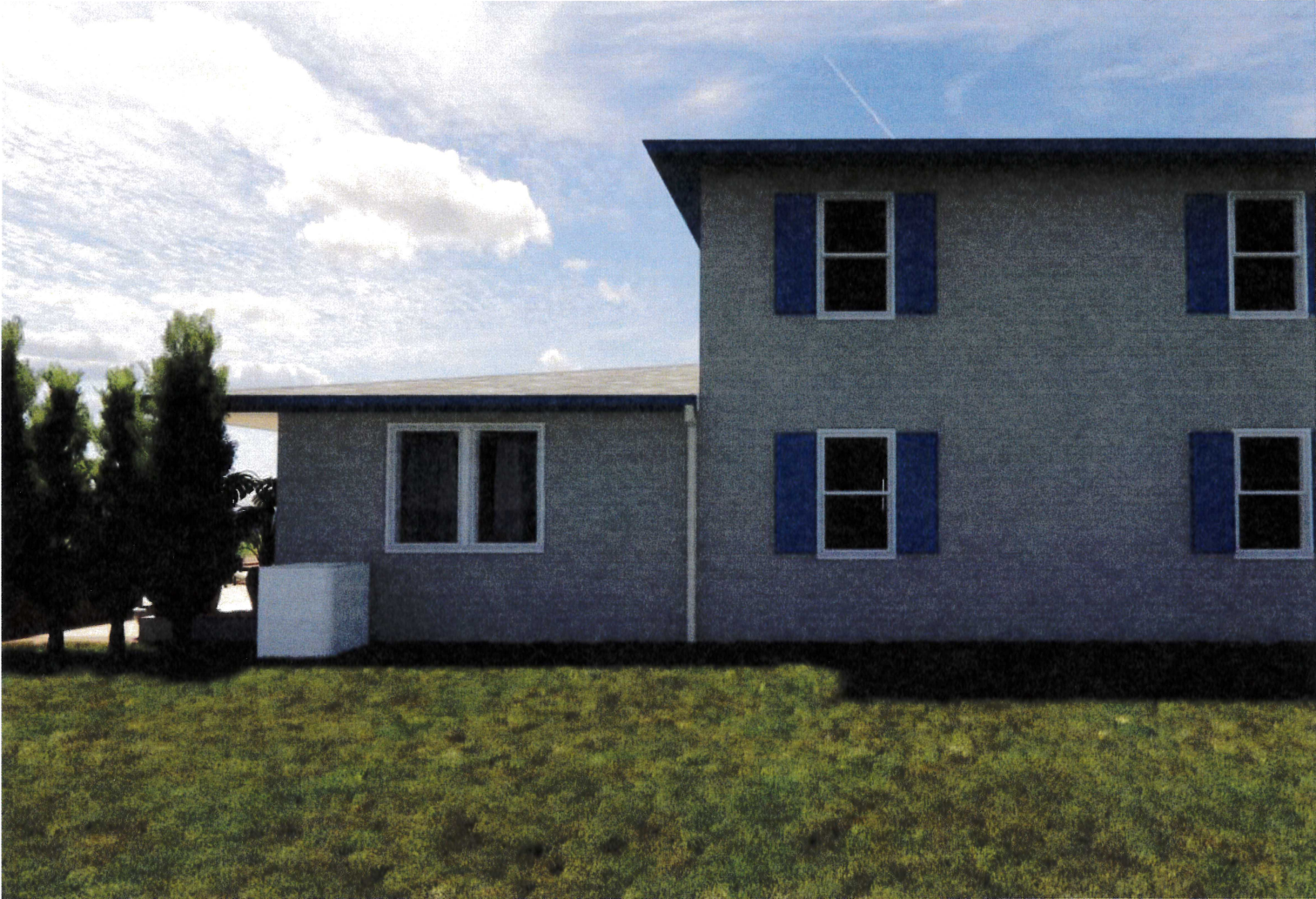
VIEW OF NORTH FACADE: REAR ADDITI
