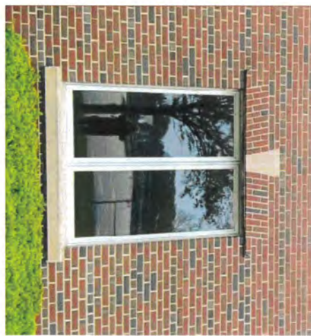
NEW: MAINTAIN PROFILE AND ADD HORIZONTAL MULLION TO MATCH REST OF WINDOWS
