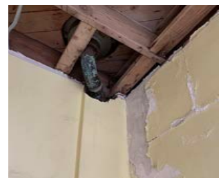
Bayside - Roof leaks lead to damaged ceilings.
