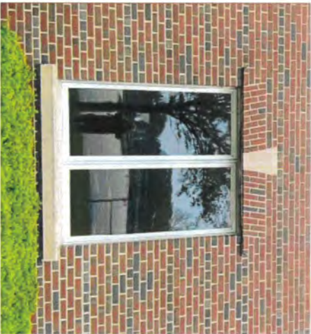
NEW: MAINTAIN PROFILE AND ADD HORIZONTAL MULLION TO MATCH REST OF WINDOWS
