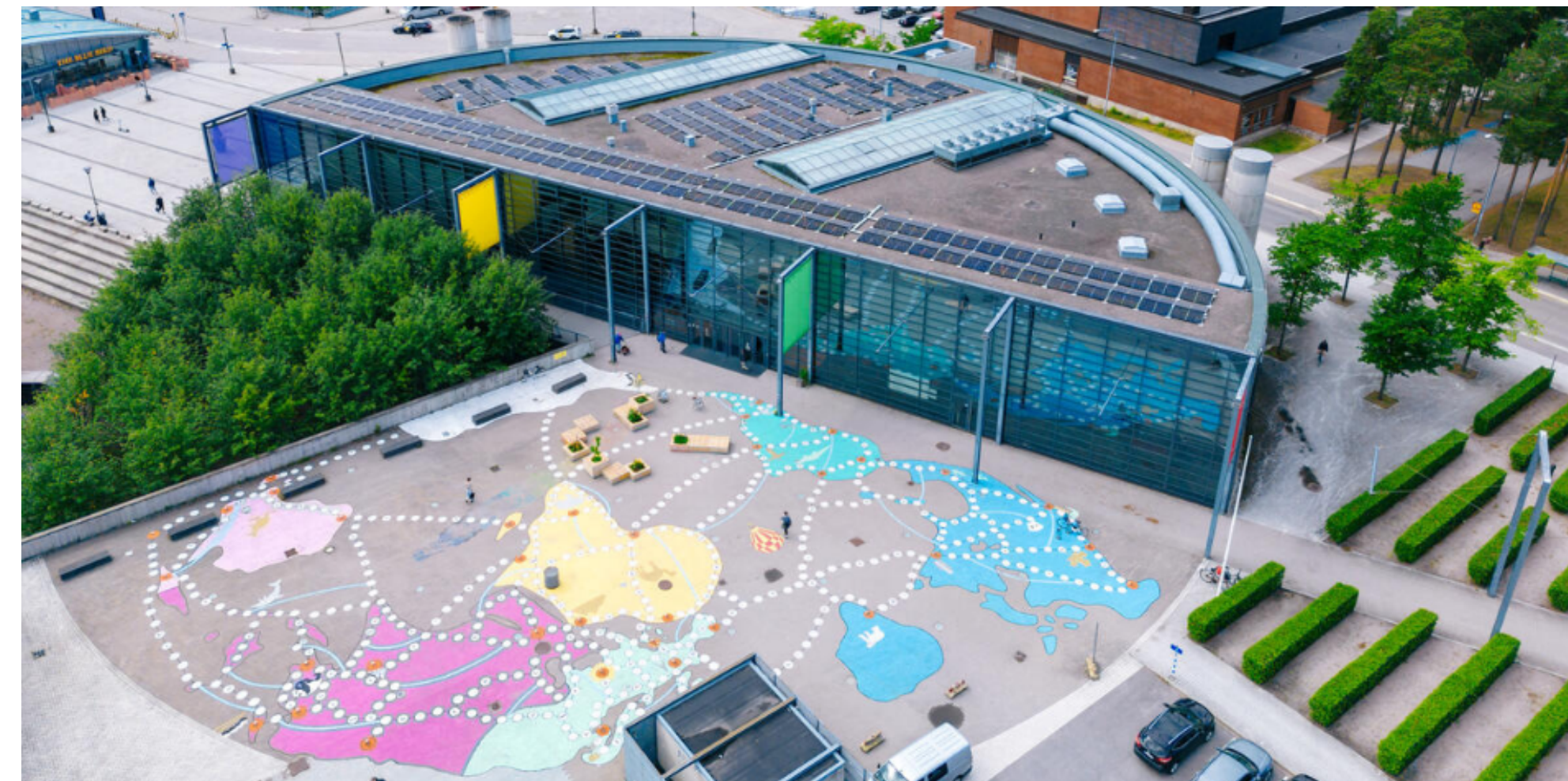
EXAMPLE OF A PAINTED TERRACE
