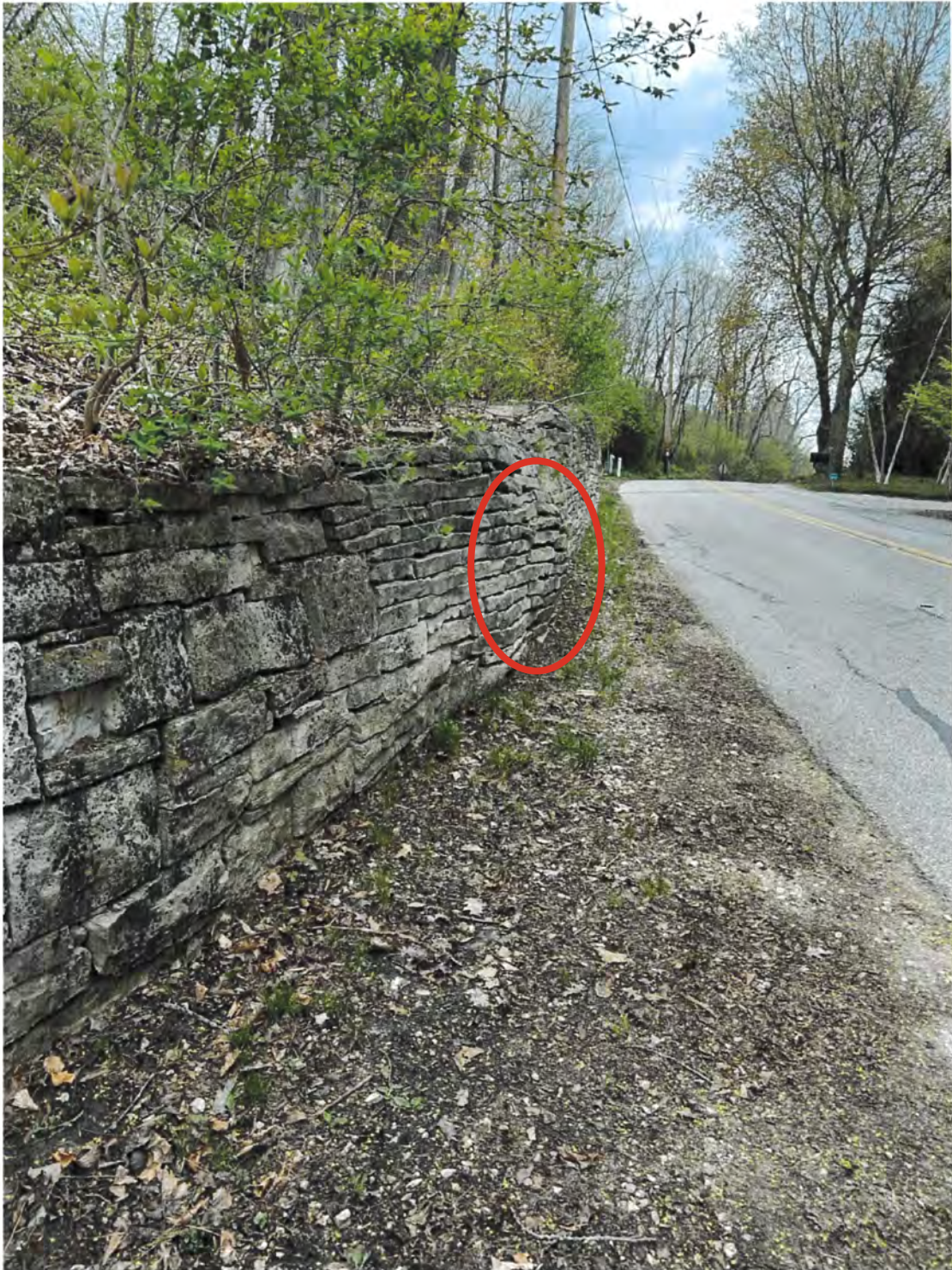
Image 3 – Retaining Wall 7900 block Beach Drive – May 2026
