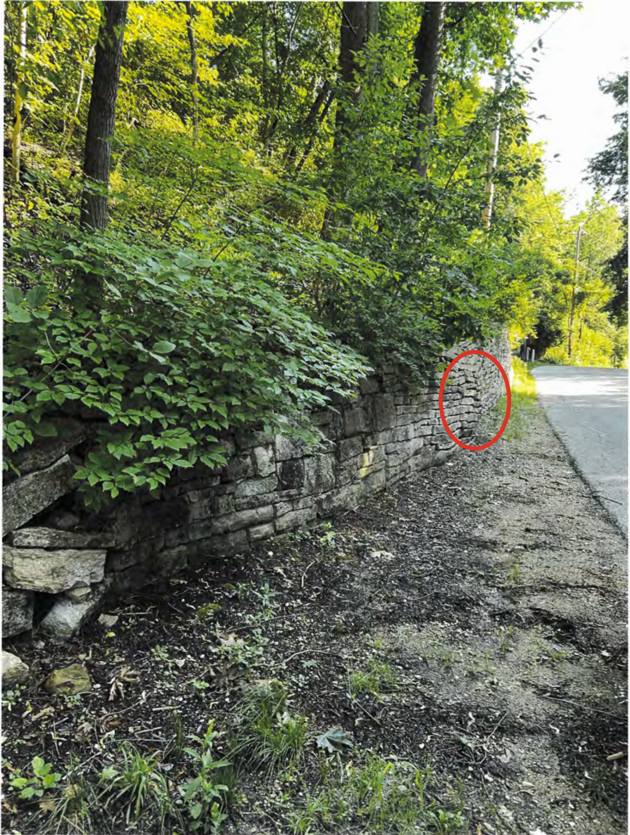
Image 2 – Retaining Wall 7900 block Beach Drive – July 2025
